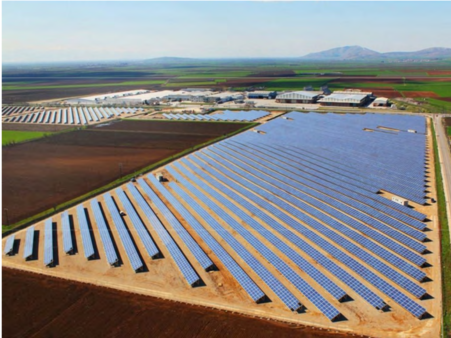
10MWp ground mounted park, Farsala
