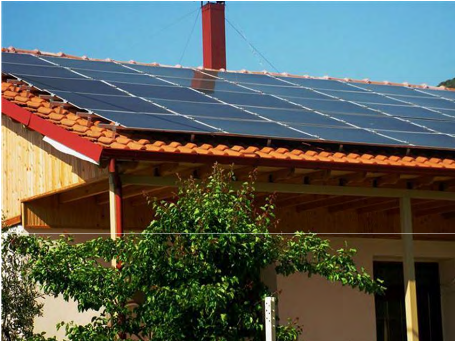
10kWp residential rooftop, Athens
