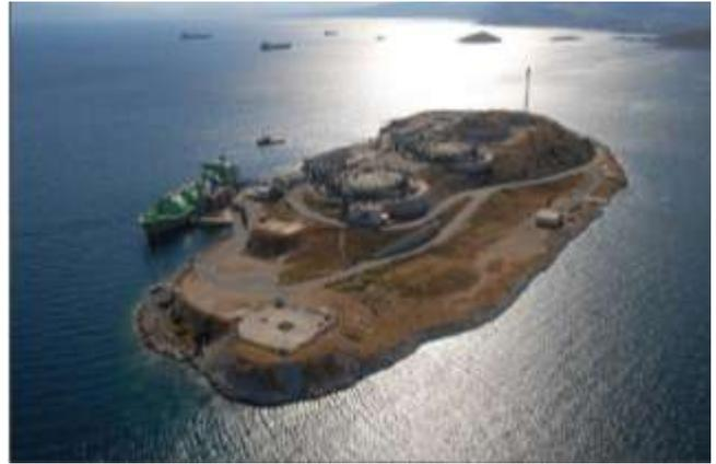
Today, the Terminal has the capacity to accept and handle some 5.2 -5.3 billion m<sup>3</sup> annually. More specifically, following an expansion of the infrastructure and upgrading of the facilities SMSR gasification capacity to 1,000 m<sup>3</sup>/h of LNG from 271 m<sup>3</sup>/h LNG previously and the peak gasification has increased its capacity to 1,250 m<sup>3</sup>/h from 500 m<sup>3</sup>/h LNG.
