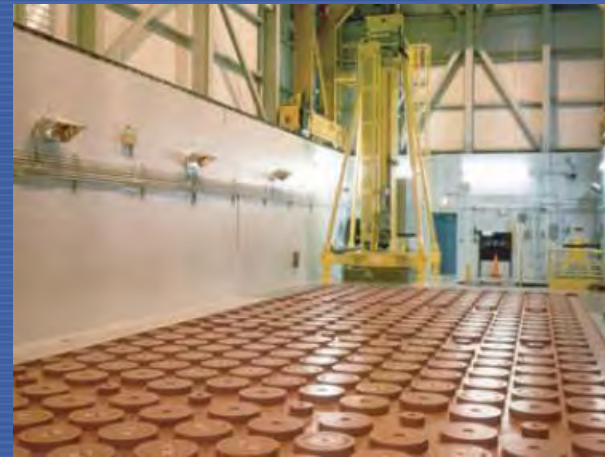
Dry storage building
