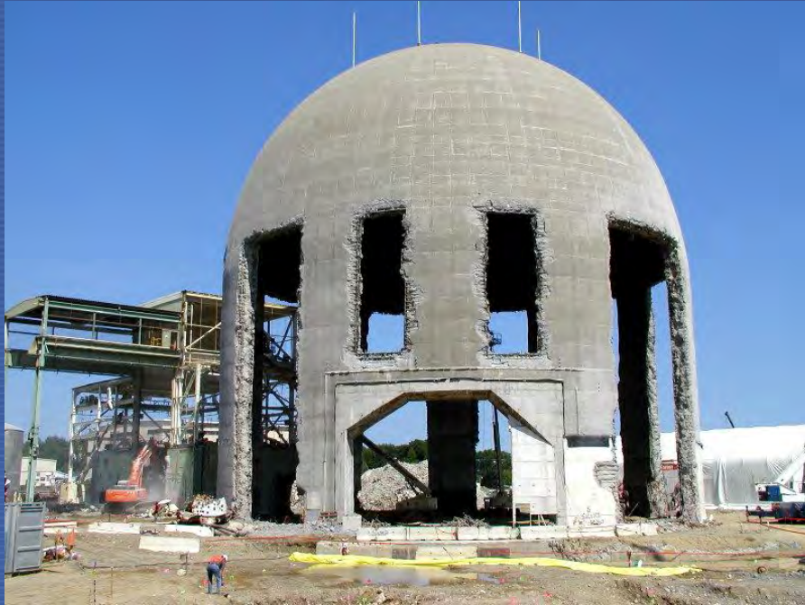
Maine Yankee being dismantled, USA
