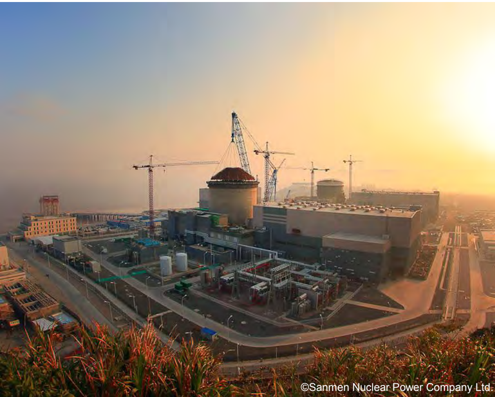
AP1000 Plant Site at Sanmen, China
